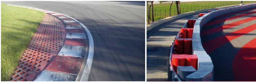
Figure 6 Inner curbs and TECPRO energy dissipation system [16, 17]
