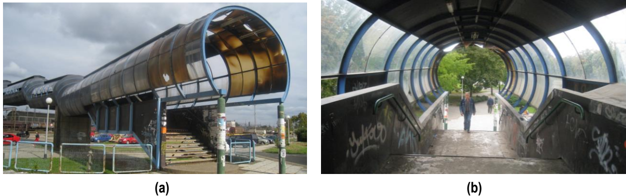
Figure 15 Pedestrian bridge at the railway station, Slavonski Brod, Croatia, authors: Duško Medaković (conceptual design and architecture), Dušan Bošnjak (construction), 1988: (a) Entry point of the pedestrian bridge on the south side; (b) Elliptical cross-section
