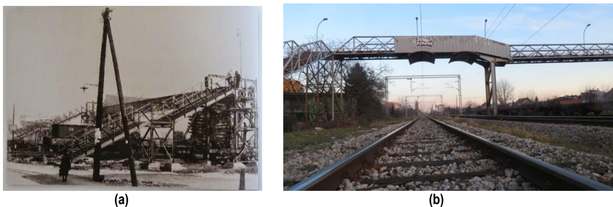
Figure 12 Pedestrian crossings over railway corridors: (a) Crossing over a railway corridor, Rural Road, Zagreb, Croatia (dismantled) [28]; (b) Crossing over a railway corridor, Kustošija city district, Zagreb, Croatia [29]
