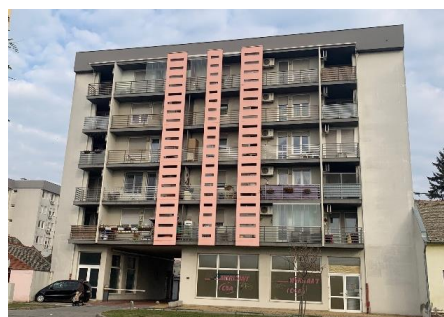
(f) A building built in the period from 2006 to 2009
