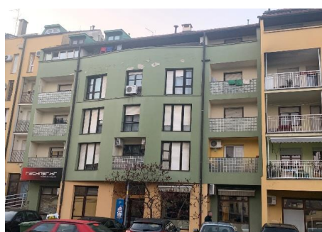
(e) A building built in the period from 1988 to 2005
