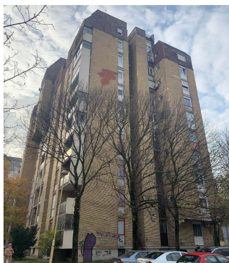
(c) A building built in the period from 1971 until 1980.
