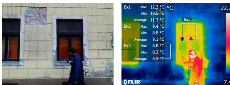
Figure 24. Termogram of Kostić house in 23 Kuhačeva Street.
