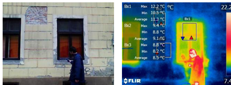
Figure 24. Termogram of Kostić house in 23 Kuhačeva Street.
