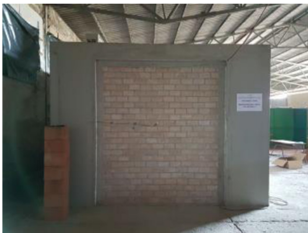
Figure 3: Wall made of concrete blocks with recycled brick aggregate.
