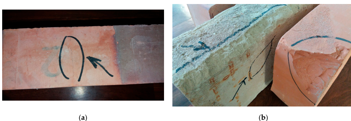
Figure 1. Typical appearance of non-resistant bricks after 25 freeze-thaw cycles, (a) damage in the form of cracking; (b) damage in the form of delamination.
