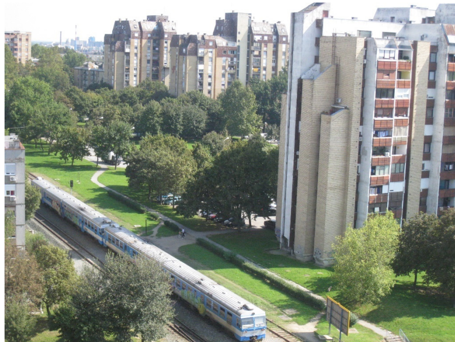
Figure 4. Conflicting linear direction of the railway and the housing estate Sjenjak in Osijek, Croatia.
