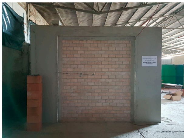
Figure 5. Wall made of RBC-EP masonry block—without isolation.
