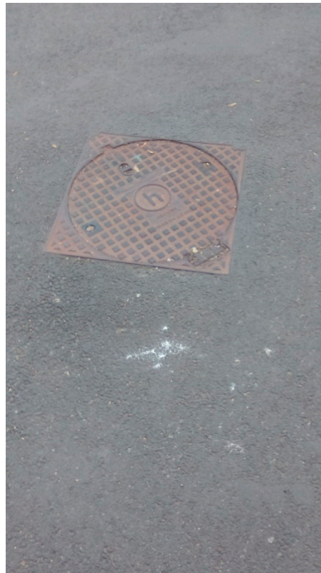
Figure 12. Manhole cover (Photo by D. Obradović).
