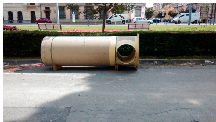
Figure 10. GRP manhole delivered for installation (Photo by D. Obradović).
