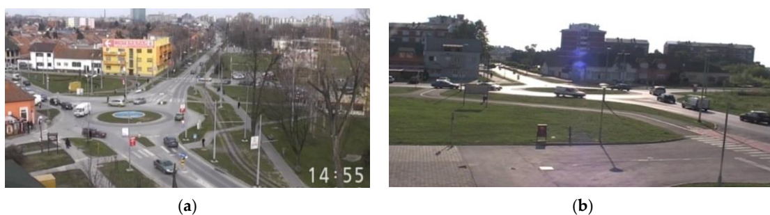
Figure 1. Observed roundabouts. (a) First roundabout; (b) second roundabout.
