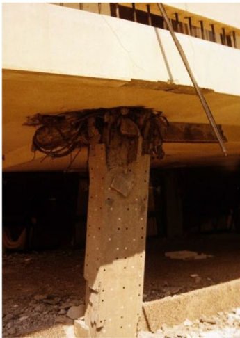
Fig. 26 Damage of the Hotel “Slavija” buildings (type RC1) in Budva due to the 1979 Montenegro earthquake: a an exterior view of the hotel before the earthquake (FOS Media 2020); b the collapsed block, and c a column damage detail (Petrović 1979)
