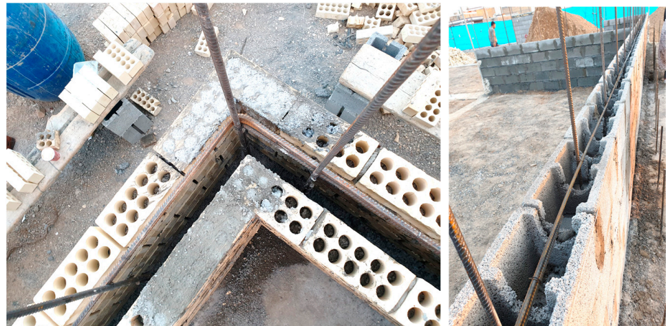
Figure 9. RM walls reinforced with steel bars, Shiraz, Iran.
