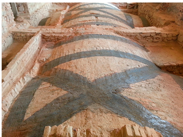
Figure 14. Vaults strengthening at the extrados [64].
