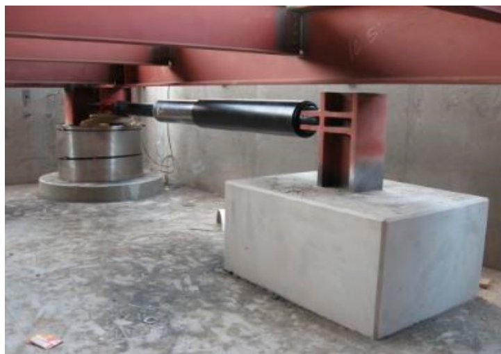
Figure 6. FVD's location in the isolated building [60].
