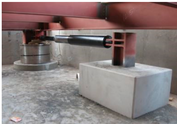
Figure 6. FVD's location in the isolated building [60].
