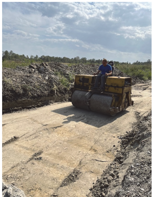
Figure 12. The compaction of the subgrade stabilized by wood ash
