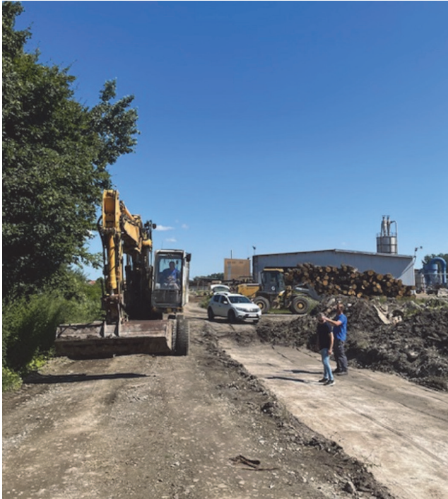
Figure 4. Planned and compacted subgrade at Test field 1
