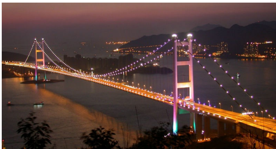
Slika 5 – Most Tsing-ma, Hong Kong
