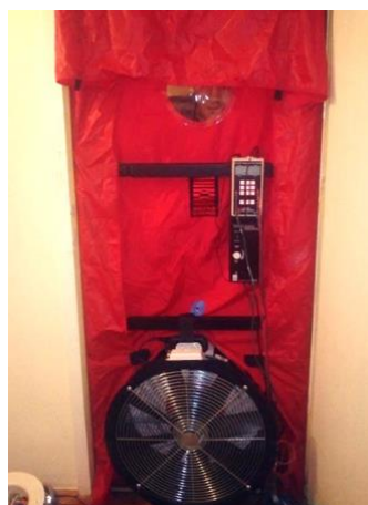
Figure 3 Blower door fan with manometer DG-700 [10]
