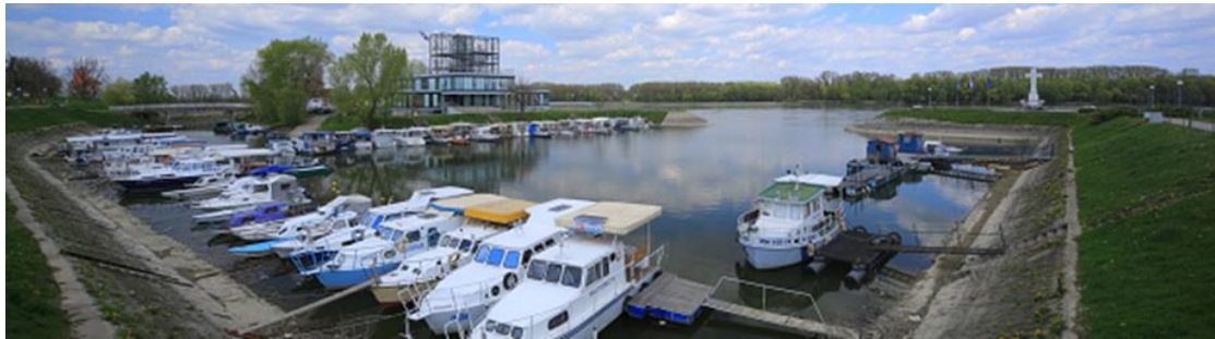
Figure 2 Winter port, special purpose port, Danube River, Vukovar
