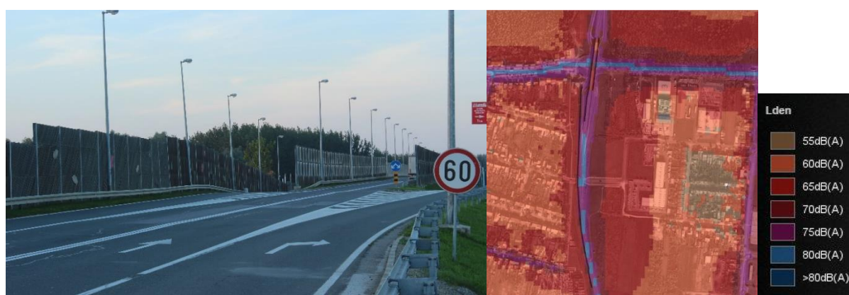
Figure 3 a) Noise barrier on west bypass and b) the effect of the noise barrier on noise levels
