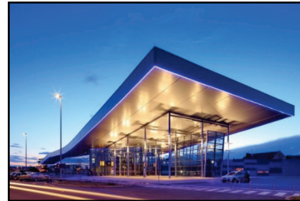
Figure 22 Bus station in Osijek (Croatia) with an aluminium-glass tramehorizontale façade type [43]
