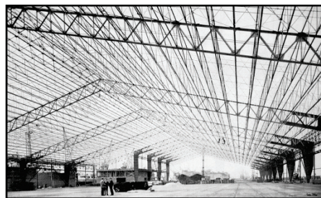
Figure 14 A frame system warehouse structure in Antwerpen [3]
