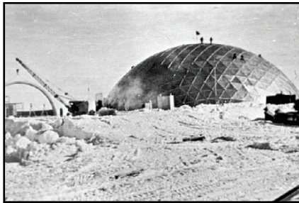
Figure 4 Aluminium dome research station in South Pole [3]
