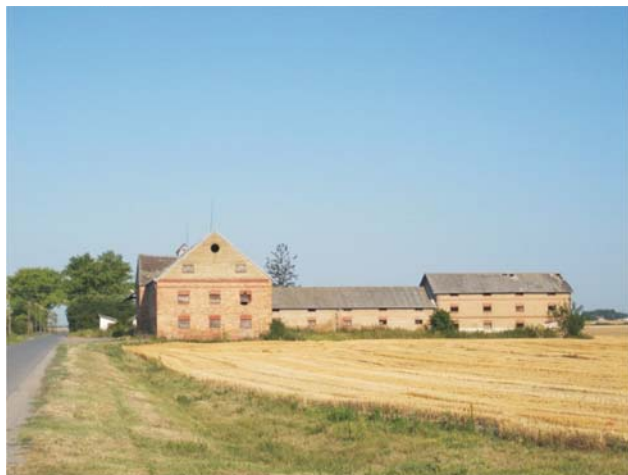
Figure 1 A planned settlement – Jasenovac Slika 1. Pustara Jasenovac
