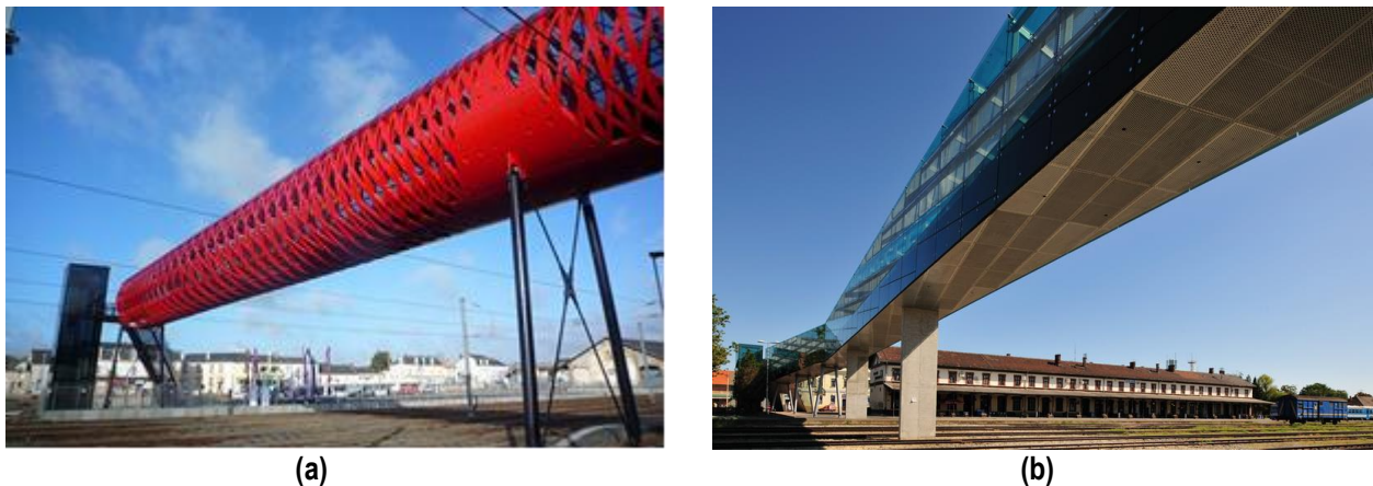
Figure 3 Linear pedestrian bridges: (a) Pedestrian bridge at the railway station, La Roche-Sur-Yon, France, architect: Bernard Tschumi, 2010 [11]; (b) Pedestrian bridge at the railway station, Osijek, Croatia, architects: Branimir Kljajić and Goran Jagić, 2009
