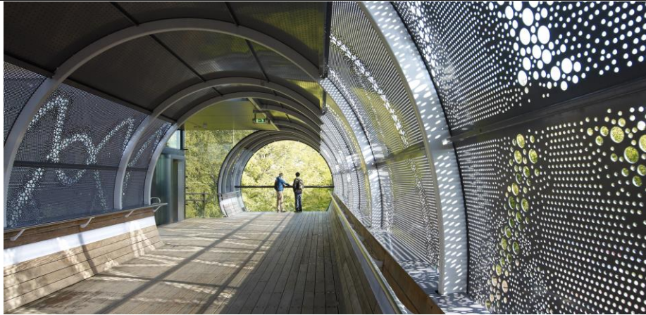
Figure 9 Circular or elliptical cross-section: Pedestrian bridge at the railway station, Hilversum, the Netherlands, architects: MVSA-architects, 2011 [23]
