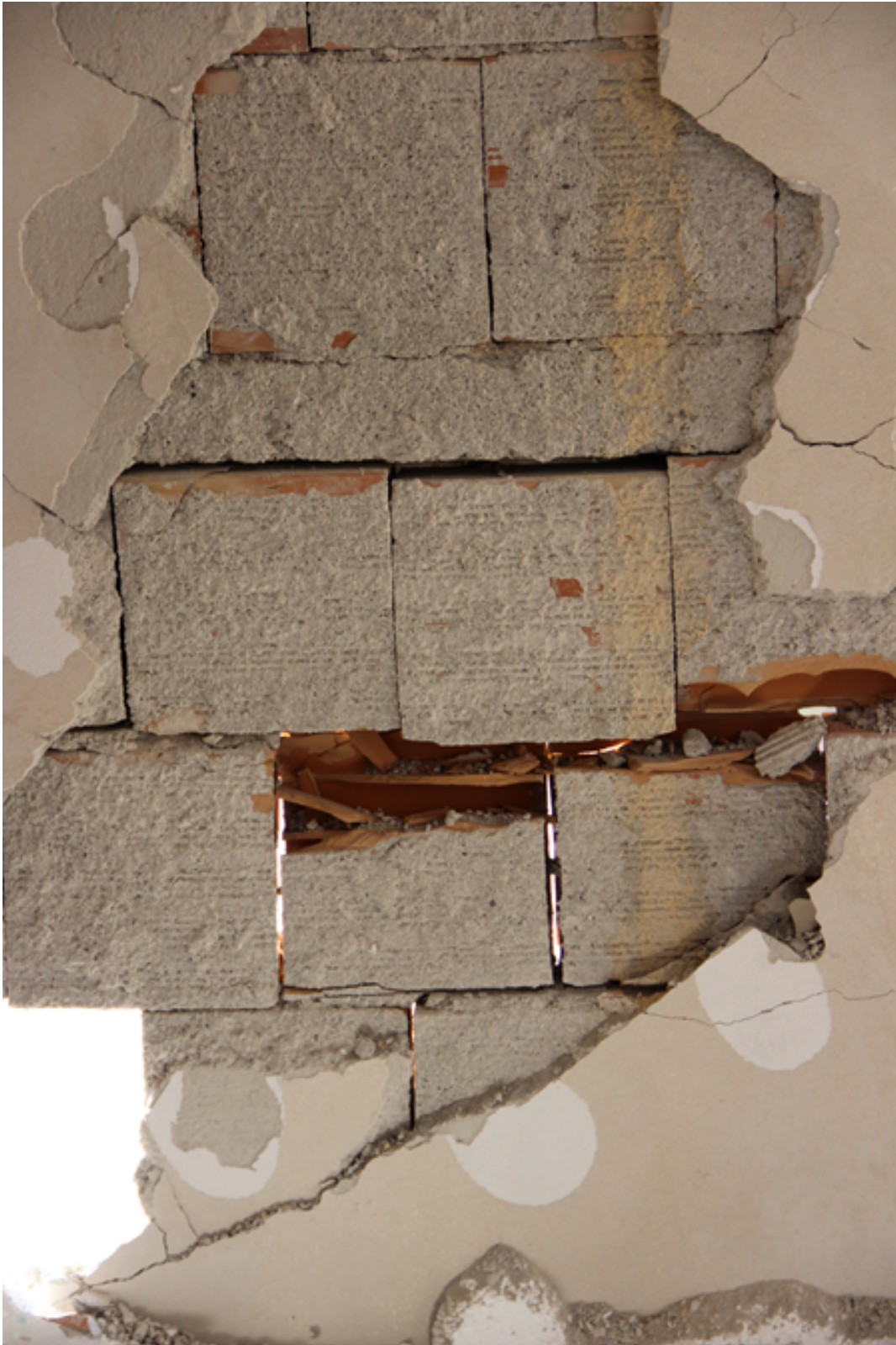
Figure 1.8: Masonry units sparsely bounded with mortar
