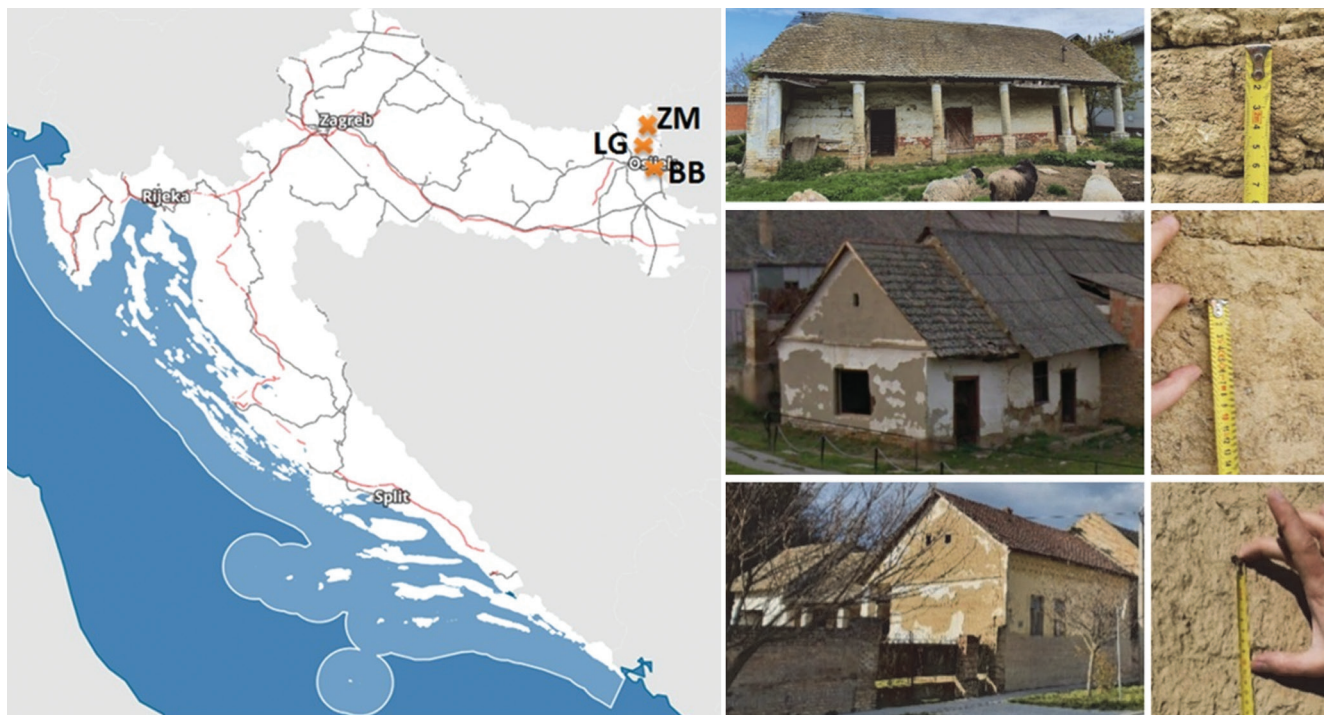
Figure 2. Position of the observed buildings on the map of the Republic of Croatia (taken from [12] and edited, left); Building BB and thickness of the compacted layer (author's photos, top right); House LG and the thickness of the compacted layer (author's photos, middle right); House ZM and the thickness of the compacted layer (author's photos, bottom right)
