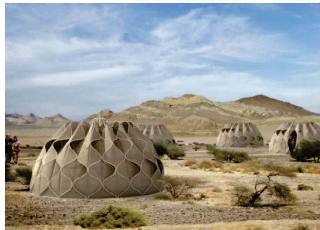
Figure 4 Temporary shelter for all the types of natural disasters, Abeer Seikaly, 2013
