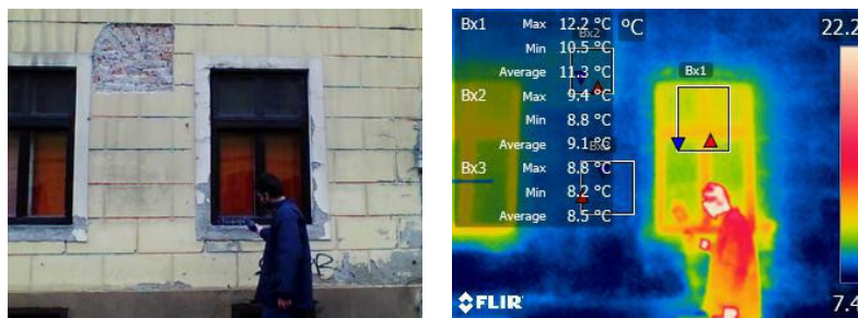
Figure 24. Termogram of Kostić house in 23 Kuhačeva Street.
