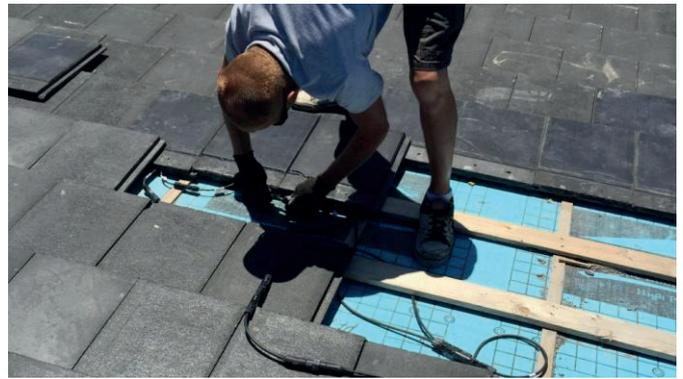
Figure 3. An integrated solar cell in roofing, [4]
