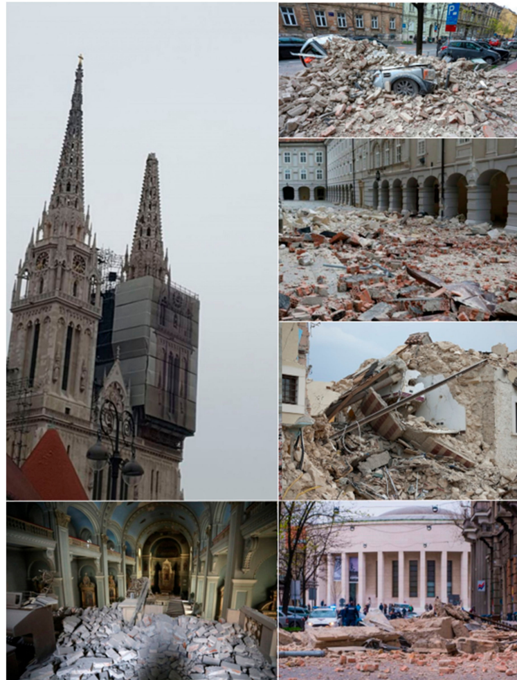
Figure 6. Photos of damage in Zagreb caused by the 22 March 2020 earthquake.
