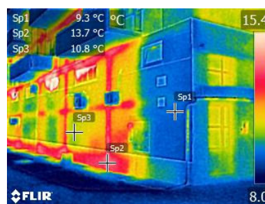
Figure 2. An example of highly-visible structural elements as well as a heated and an unheated space.
