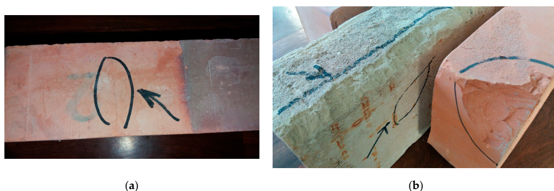
Figure 1. Typical appearance of non-resistant bricks after 25 freeze-thaw cycles, (a) damage in the form of cracking; (b) damage in the form of delamination.
