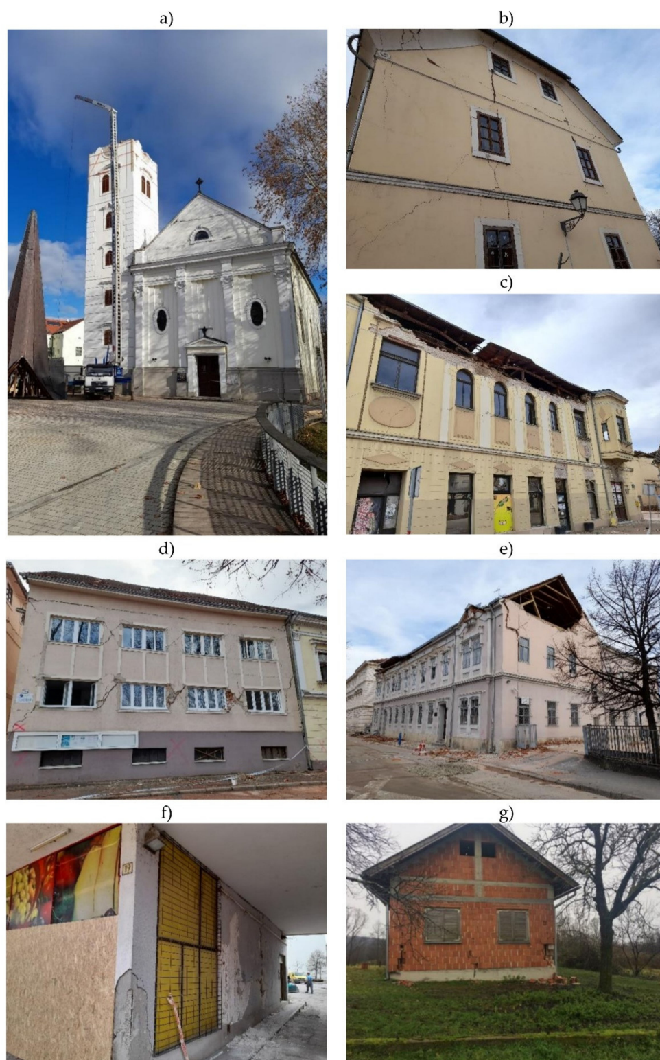
Figure 11. Damages that were sustained by various building types built in the pre-code era (before 1964) and in various code eras: (a) The Cathedral of the Exaltation of the Holy Cross in Sisak with the tower roof removed; (b) Crack distribution in an old masonry building in Petrinja; (c) Parapet wall collapse in an old masonry building in Petrinja; (d) Masonry pier diagonal tension cracking; (e) Gable wall out-of-plane collapse in an elementary school in Petrinja; (f) Damage to the masonry-infilled RC frame (soft storey collapse); and (g) Damage to a building that was built without vertical confining elements as part of a rebuilding programme in the post-war era [58] (author of all photos: D. Penava).
