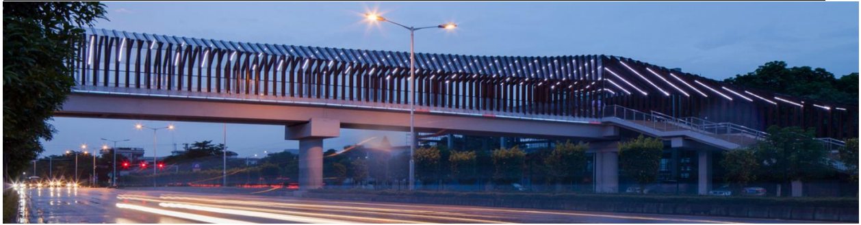
Figure 7 Pedestrian bridge over a road, Foshan, China, architects: ADARC Associates, 2015 [20]
