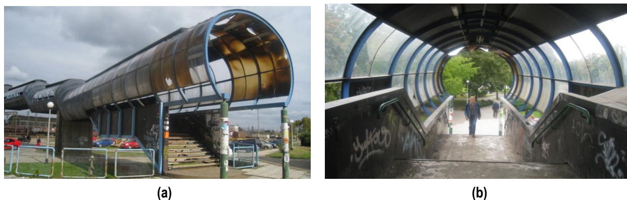
Figure 15 Pedestrian bridge at the railway station, Slavonski Brod, Croatia, authors: Duško Medaković (conceptual design and architecture), Dušan Bošnjak (construction), 1988: (a) Entry point of the pedestrian bridge on the south side; (b) Elliptical cross-section
