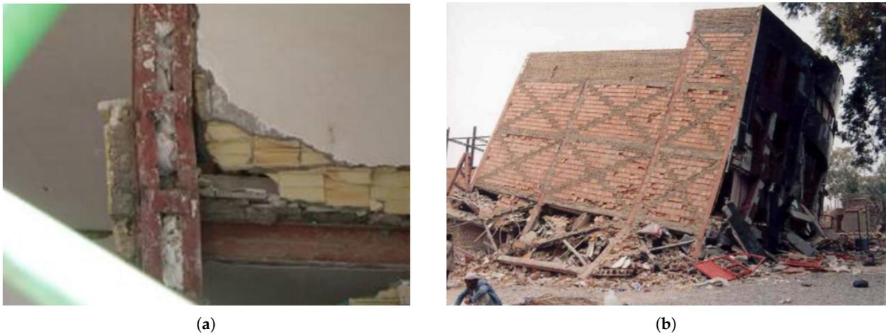
**Figure 6.** Other types of failures in structural systems [34]; (a) buckling of a column in ground floor connected to the balcony beam; (b) inappropriate lateral bracing system and longer length of first floor column led to a soft story building.
