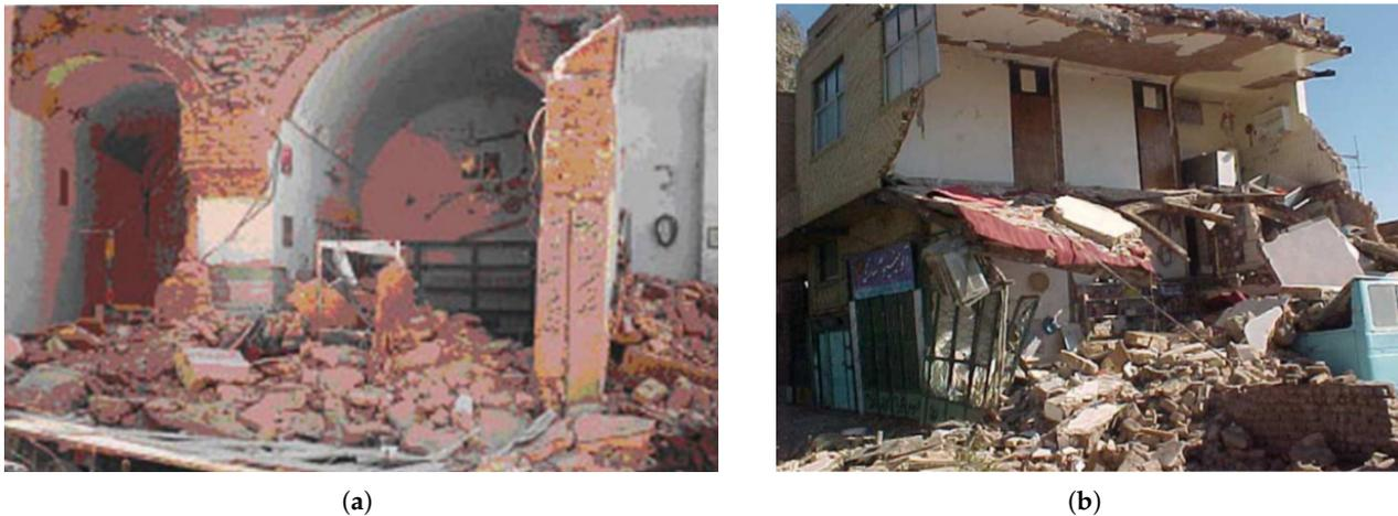
**Figure 4.** (a) Partially damaged old masonry buildings' arch roofs in Bam after the earthquake [31]; (b) the inconsistency of the multi-arched roof with the supports due to the lack of horizontal coils, as well as the high thickness and weight of the roof [31].
