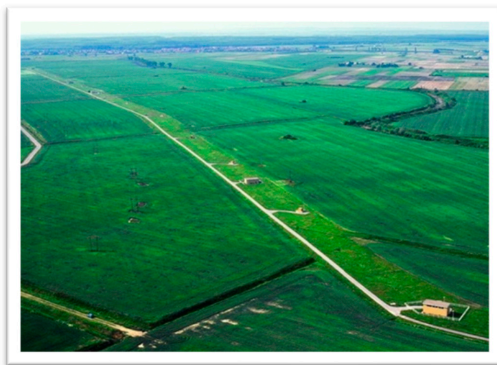
Figure 4. Photograph of the Vinogradi Pumping Station, Osijek, Croatia (Fund of documents of the company “Vodovod Osijek, Osijek, Croatia” 2000).
