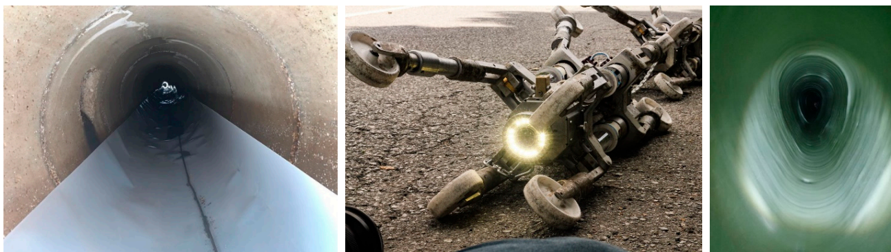
Figure 13. Renewal method—the CIPP method. Adapted with permission from ref. [102]. Copyright 2022 Solmex d.o.o.
