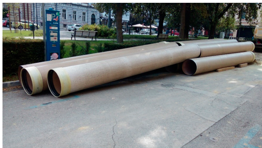
Figure 8. Sewer pipes delivered for installation (Photo by D. Obradović).
