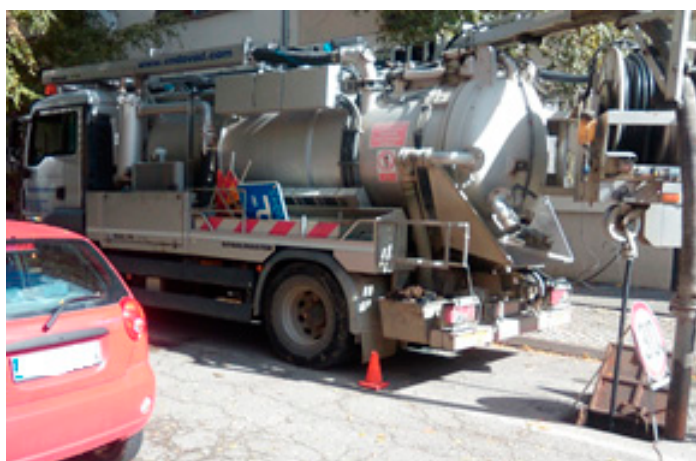
Figure 5. Sewer cleaning truck (Photo by D. Obradović).
