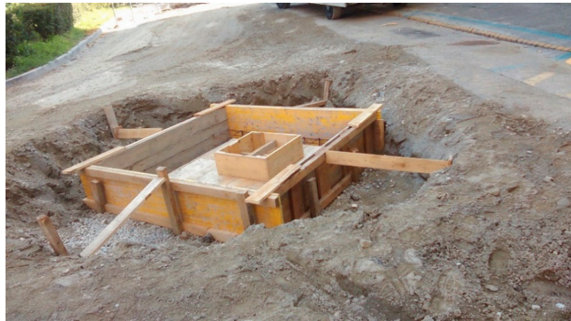
Figure 7. Formwork for sewer control shaft—manhole (Photo by D. Obradović).
