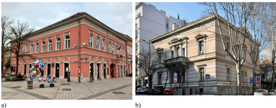
Fig. 10 URM buildings with flexible diaphragms: a type M1: an URM building with adobe walls constructed at the beginning of the nineteenth century in Dunavska Street 2, Novi Sad and b Type M2: an URM house with brick masonry walls constructed in Belgrade in 1884
