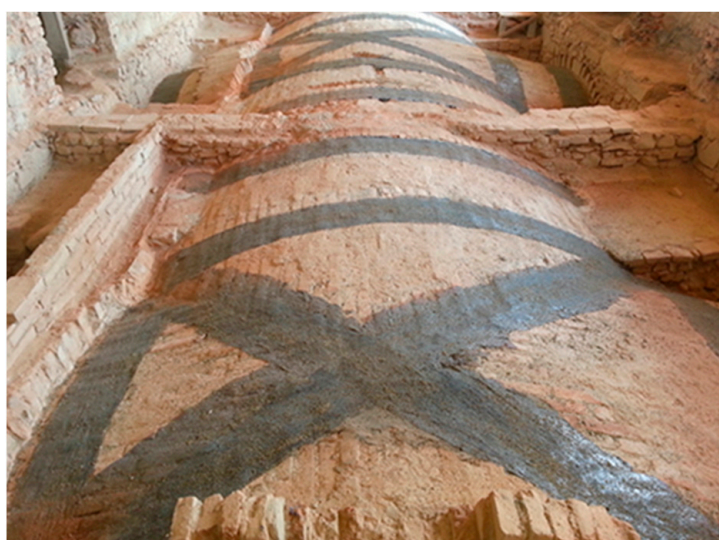
Figure 14. Vaults strengthening at the extrados [64].
