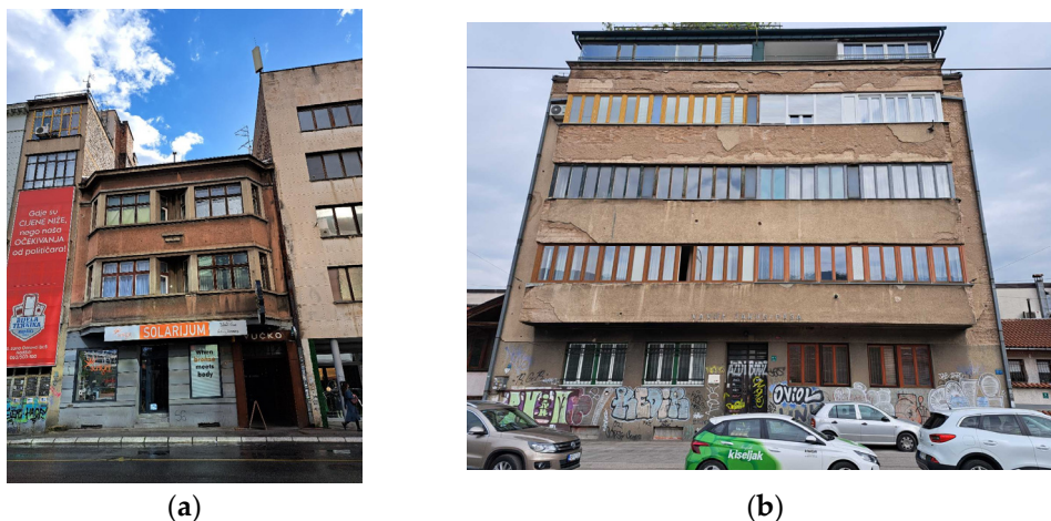
Figure 1. (a) Damić House (author’s source); (b) Jakub-Paša Building, Obala Kulina bana Street (author’s source).
