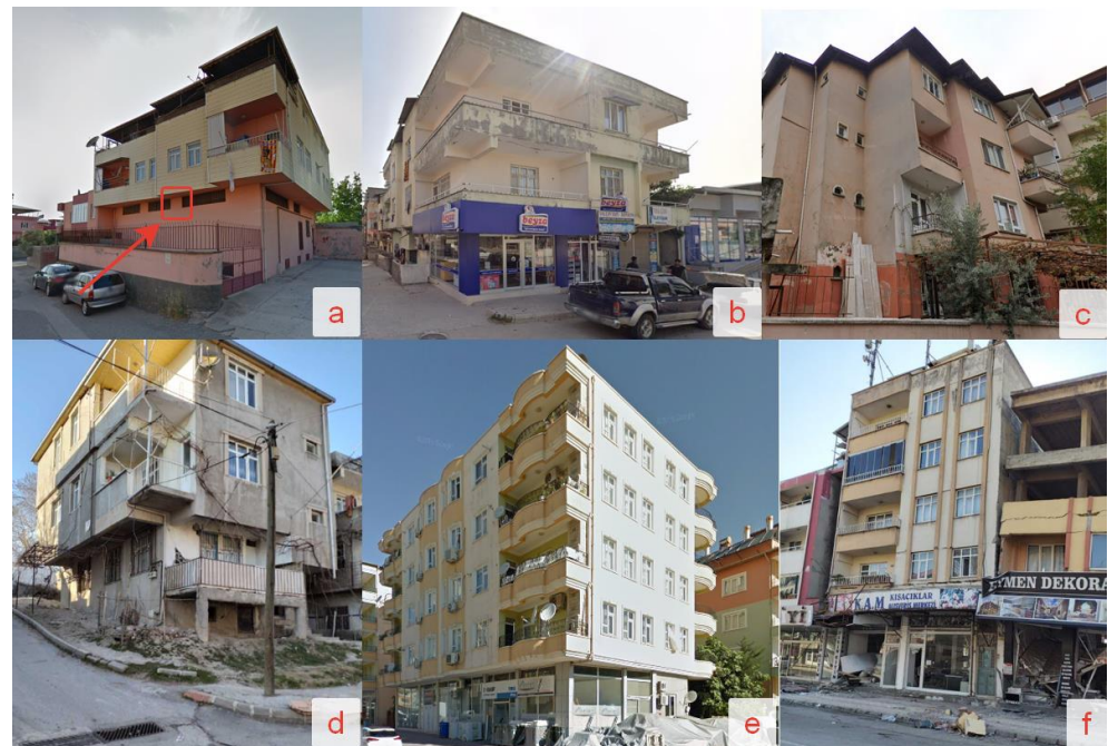
Figure 11. (a) Short column, (b) soft/weak storey, (c) plan irregularity, (d) hill/slope effect, (e) heavy overhang, (f) adjacent buildings.
