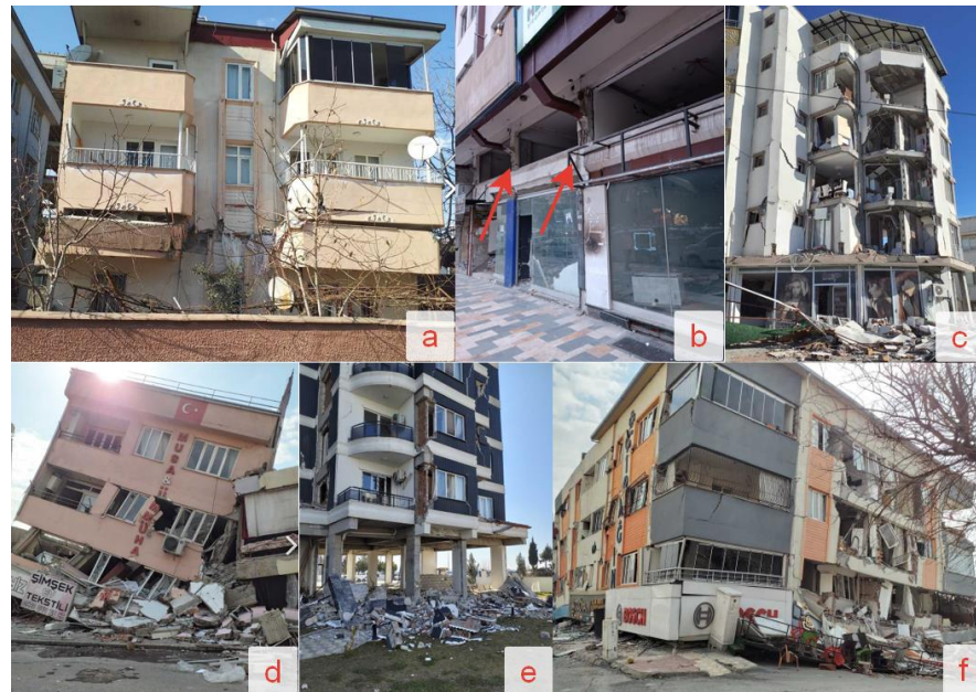
Figure 13. (a) Soft/weak-storey damage caused by mezzanine, (b) structural damage caused by short column, (c) example of damage caused by irregularity in plan, (d) example of damage caused by collision, (e) example of damage caused by heavy overhangs, (f) soft/weak-storey damage example caused by ground story.
