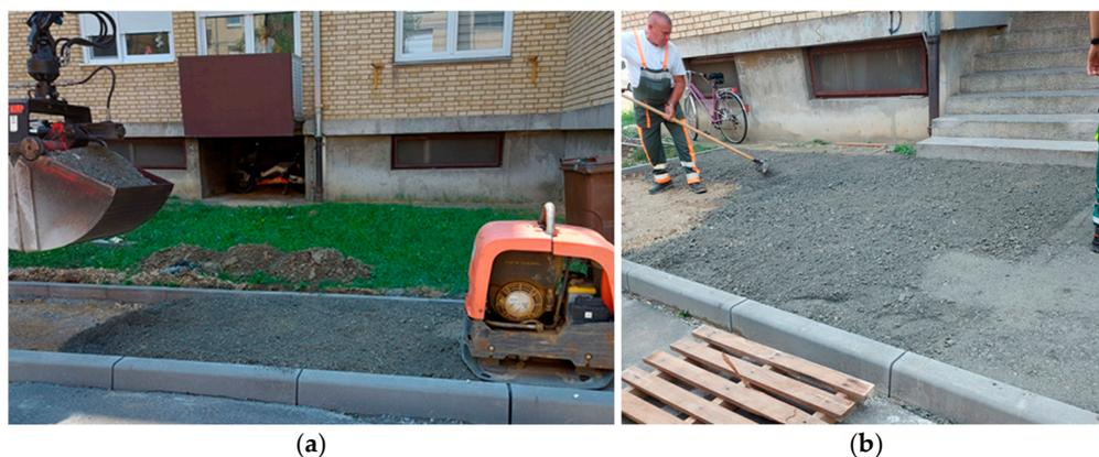
**Figure 5.** Cement-bound base layer construction: installation equipment (a) and manual spreading (b).
