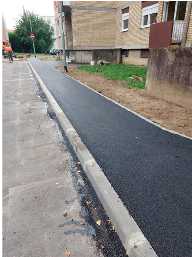
Figure 7. Completed test section.
