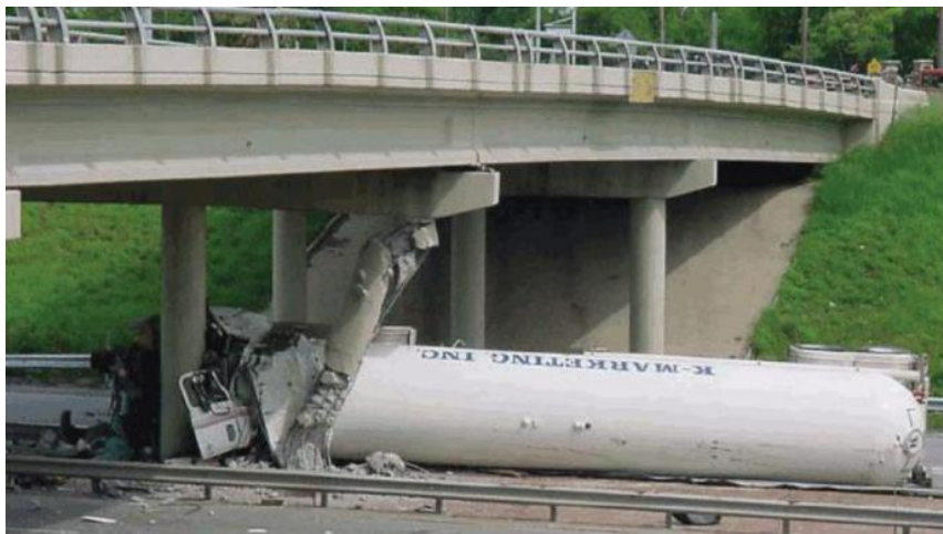
Figure 1 Impact between vehicle and column (U.S. highway) [8]
