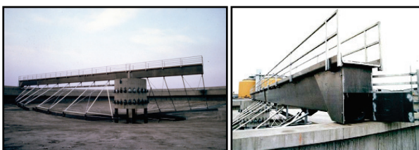
Figure 6 Rotating crane bridge in a sewage treatment plant [15]
