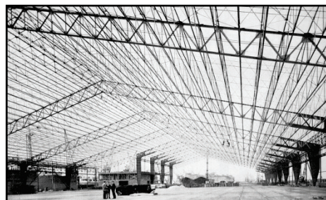
Figure 14 A frame system warehouse structure in Antwerpen [3]
