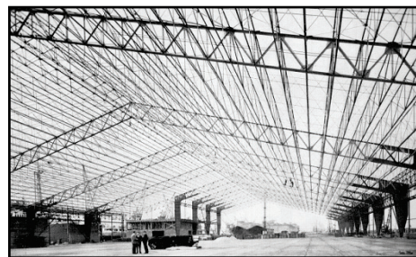
Figure 14 A frame system warehouse structure in Antwerpen [3]
