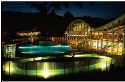
Figure 20 Tramehorizontale façade type for a swimming pool structure in Sv. Martin (Croatia) [43]
