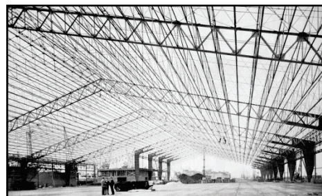
Figure 14 A frame system warehouse structure in Antwerpen [3]
