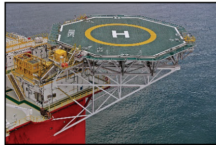
Figure 7 Aluminium helideck on an offshore platform [36]
