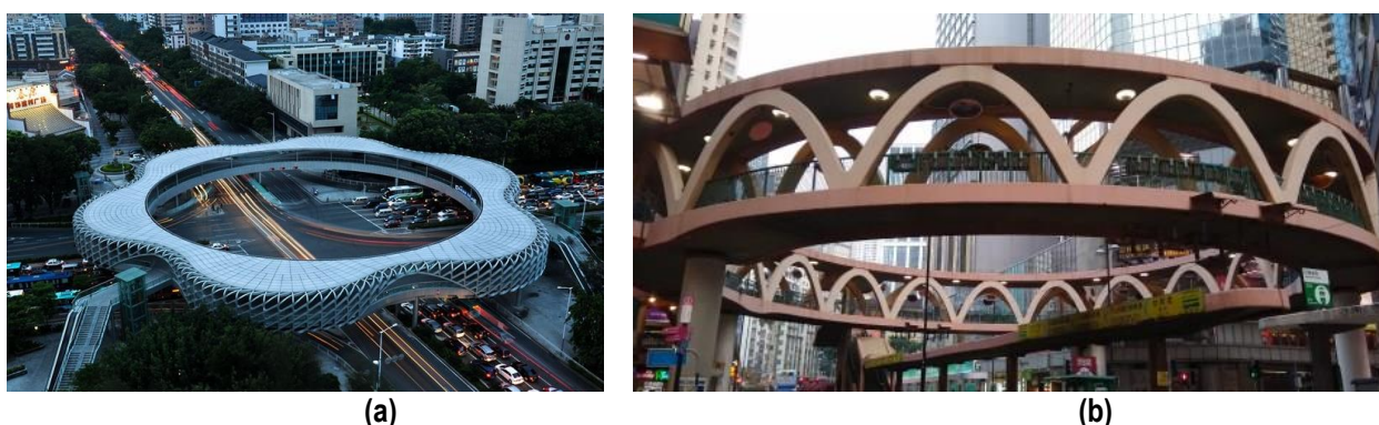
Figure 4 Circular pedestrian bridges: (a) Pedestrian bridge over an intersection, Shenzhen, China, 2012 [12]; (b) Pedestrian bridge over an intersection, Hong Kong, China [13]
