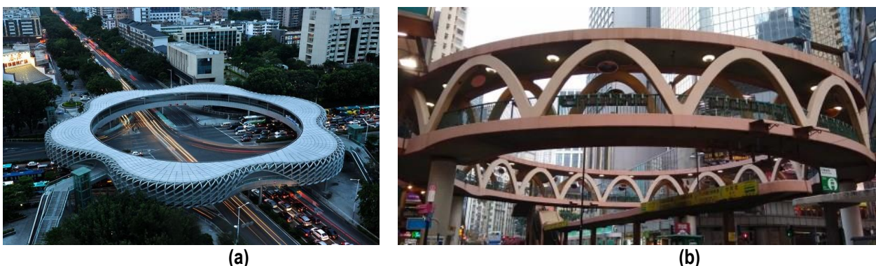
Figure 4 Circular pedestrian bridges: (a) Pedestrian bridge over an intersection, Shenzhen, China, 2012 [12]; (b) Pedestrian bridge over an intersection, Hong Kong, China [13]
