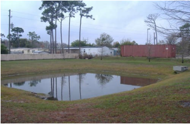
Fig. 3 Stormwater retention pond. (Source: Lapin Services, 2015).
