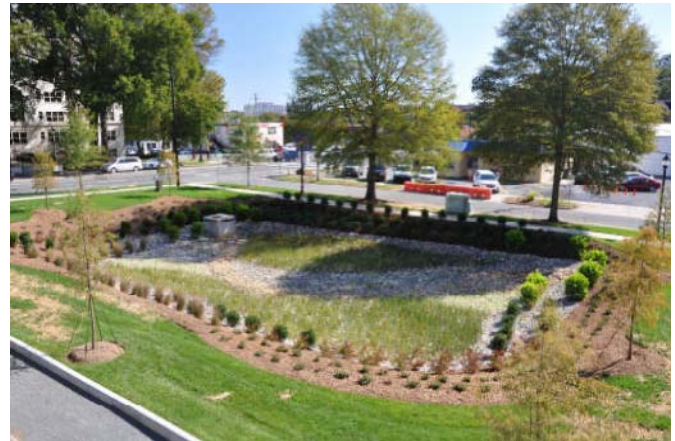
Fig. 4 Stormwater detention pond. (Source: Metrolina Landscape, 2015).
