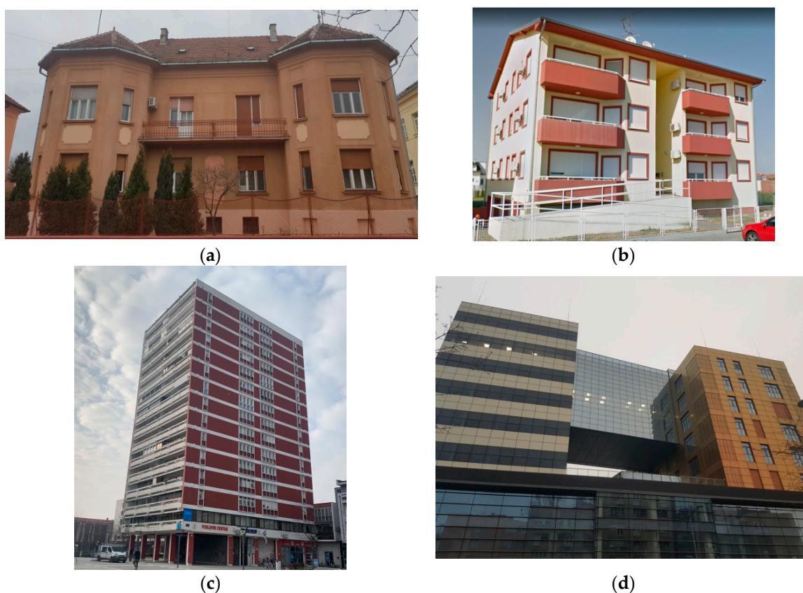
Figure 5. Typical examples of (a) older masonry buildings (with wooden floors), (b) confined masonry, (c) reinforced concrete (RC) frames, and (d) newer RC frames.
