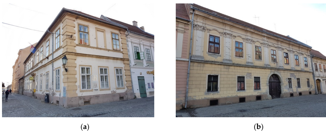
Figure 14. Kostić house (a) at the corner of Kuhačeva and Marković street (2 Markovičeva Street) and (b) in 23 Kuhačeva Street.
