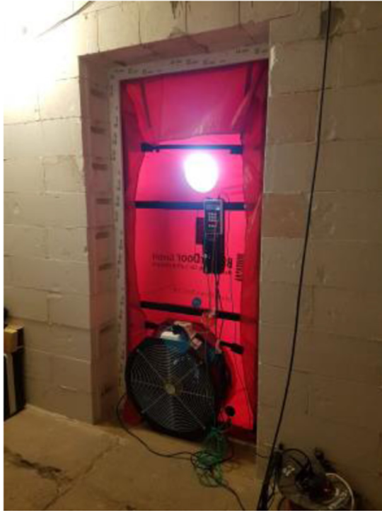
Figure 4: Blower door equipment.
