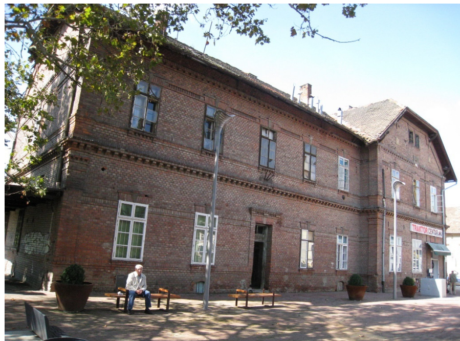
Figure 7. Historic Gutmann Narrow Gauge Railway Station today-east façade.
