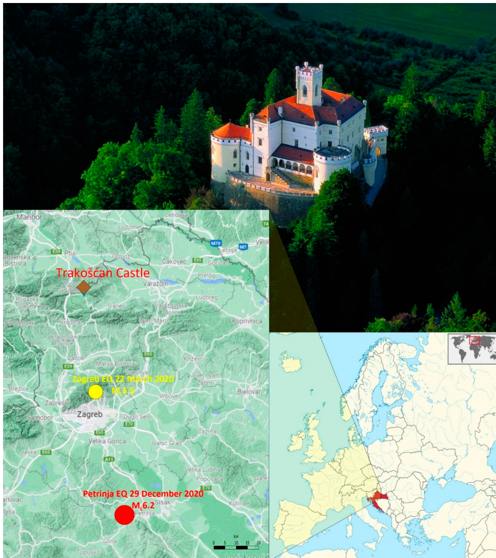
Figure 1. Photo and locations of Trakošćan Castle, and locations of the Zagreb March 2020 and the Petrinja December 2020 earthquakes.
