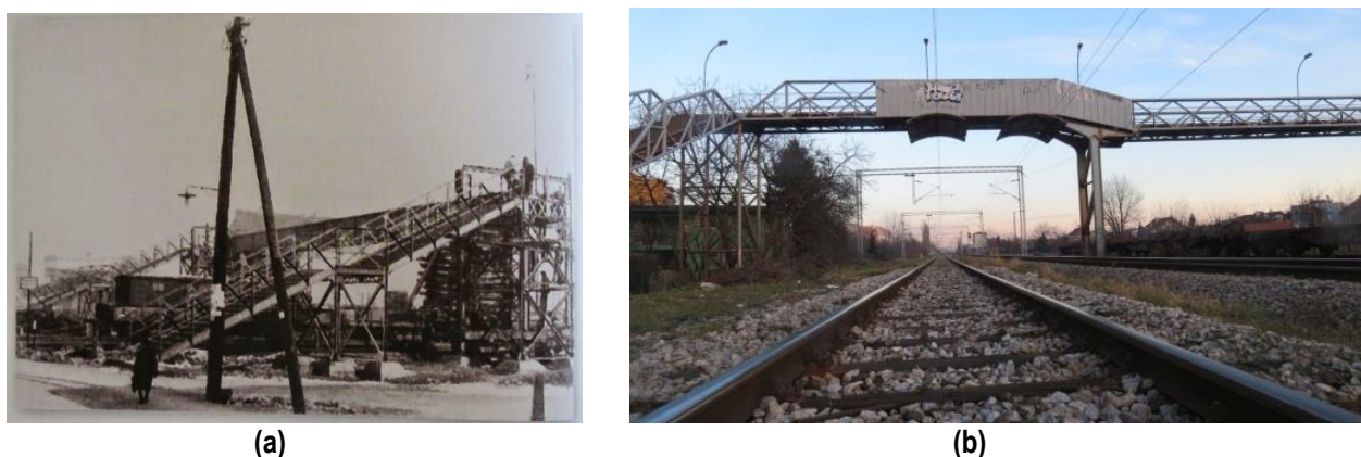
Figure 12 Pedestrian crossings over railway corridors: (a) Crossing over a railway corridor, Rural Road, Zagreb, Croatia (dismantled) [28]; (b) Crossing over a railway corridor, Kustošija city district, Zagreb, Croatia [29]
